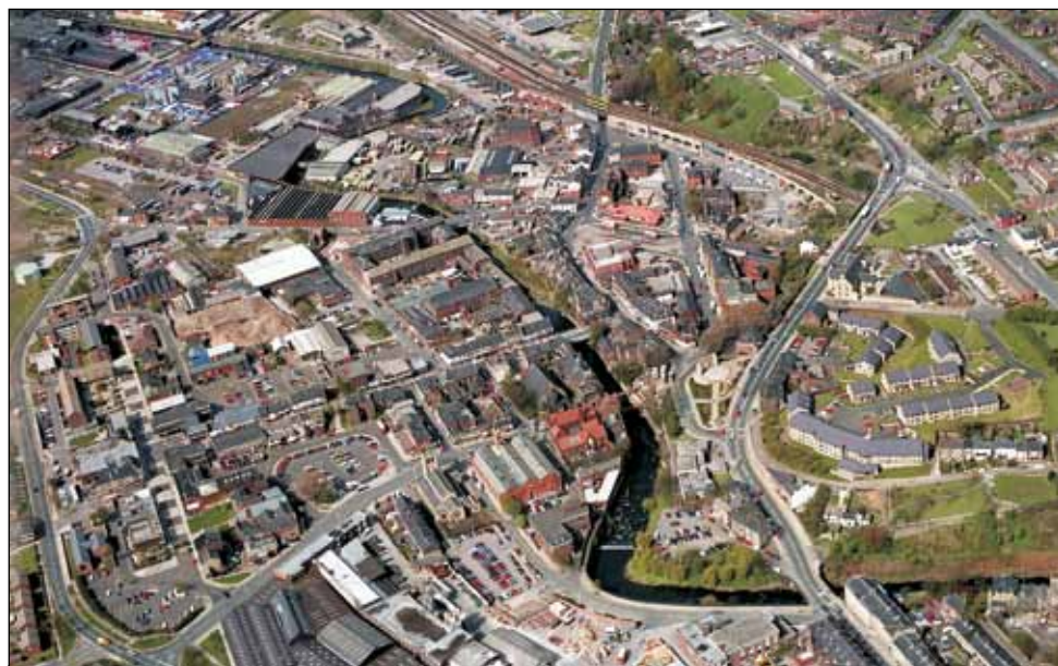
April 1991 and a high level view of Stalybridge town centre at a time when a river route for restoring the Canal was a serious option.
