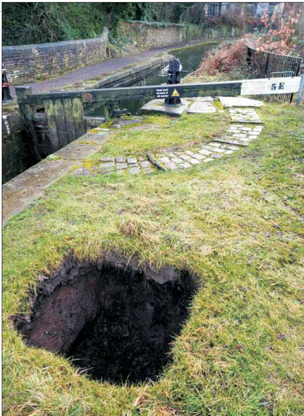
A large void appearing on the offside of Lock 5E. Leakage through the aqueduct is thought to be part of the cause. The hole is now filled, but the root problem needs investigating.
