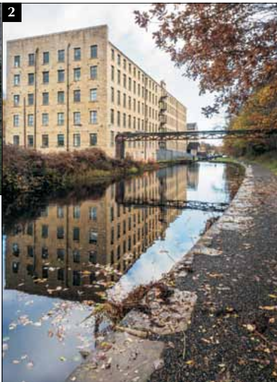
2 - Mooring rings would have been useful upstream of the lock landing stage in this location above Lock 6E. Here the Flexipave reaches the back of the wash-wall leaving no room for mooring pins.
