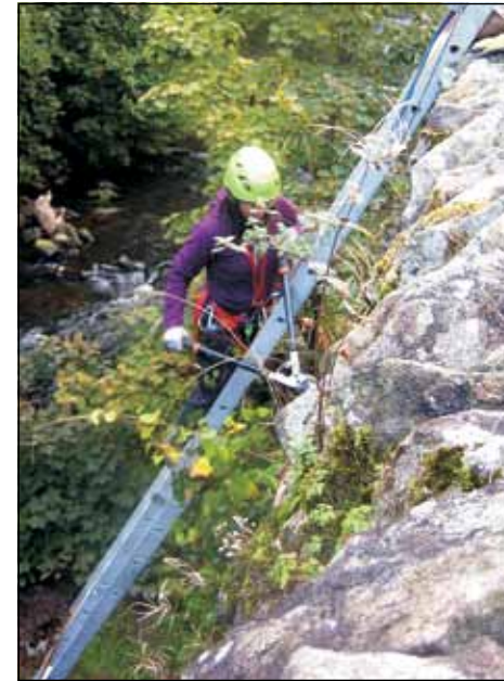
Cutting trees in the retaining wall
