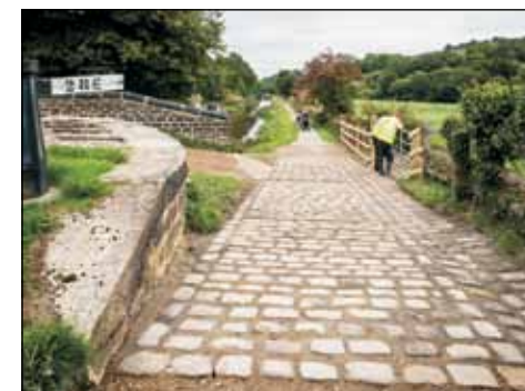
Lock 28E has the added complication of a farm accommodation bridge over the lock tail. This has meant the setts have been laid to a fall towards the field with a channel then taking any water across the ramp to the canal at the bottom. Sensibly a new gate has been fitted to allow direct access to the field without traversing a length of towpath. CRT staff admire their handy work.
