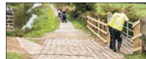
Lock 28E has the added complication of a farm accommodation bridge over the lock tail. This has meant the setts have been laid to a fall towards the field with a channel then taking any water across the ramp to the canal at the bottom. Sensibly a new gate has been fitted to allow direct access to the field without traversing a length of towpath. CRT staff admire their handy work.
