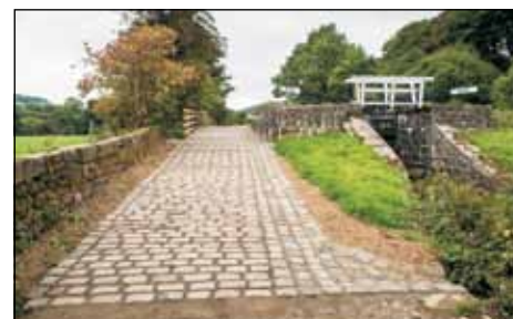
Recovered stone setts laid on the ramp at Lock 27E by the CRT construction team.
