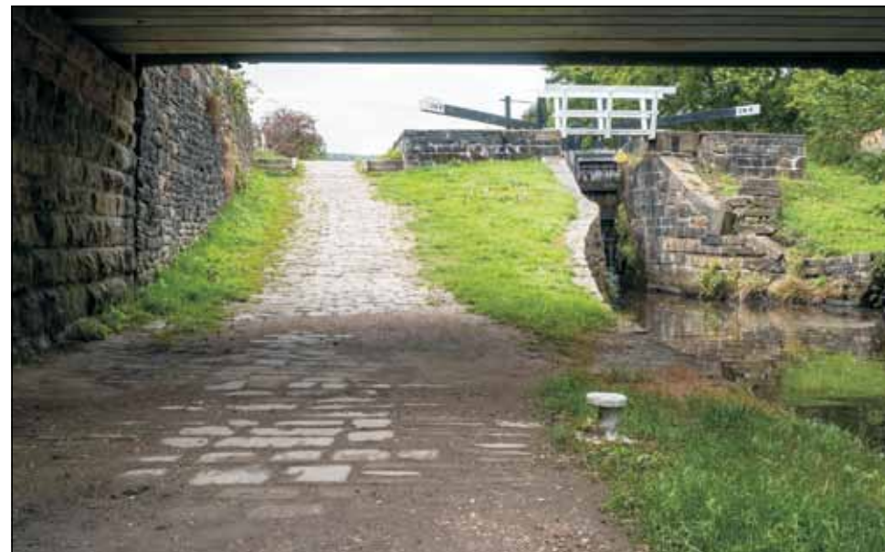
A rare surviving lock ramp retaining sandstone setts is under the bridge at Lock 29E, (September 2018).
