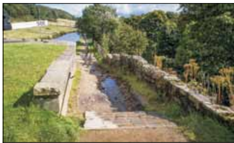
View down Lock 30E ramp in September 2012 showing severe erosion. A temporary repair was subsequently made using crushed stone.
