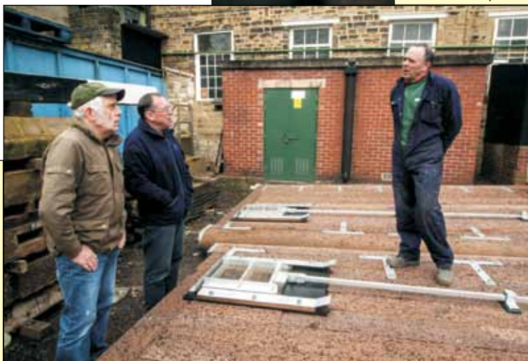
Head gates laid out in the workshop.
