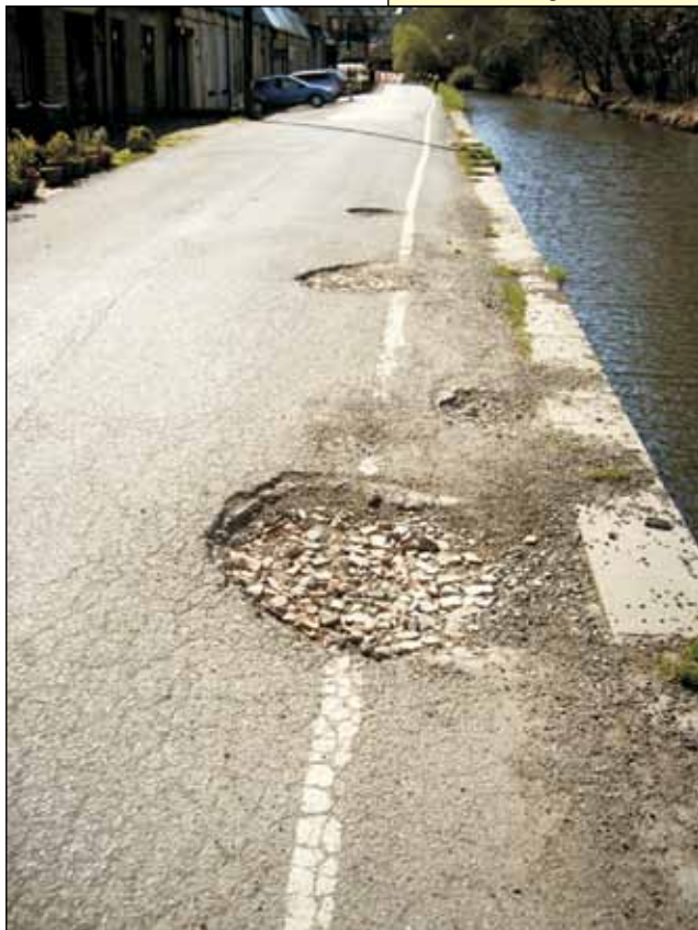
The access road in Slaithwaite suffering deterioration
