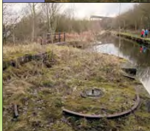
The remains of a bearing plate for the former swing bridge at Grove Road, Millbrook.
