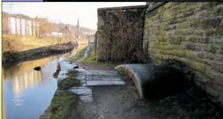
Fisher's Culvert as seen from the towpath. The substantial arched stone was installed when the viaduct was erected, protecting the culvert below.
