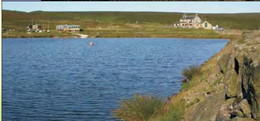
Brun Clough reservoir on Standedge Moor. It was constructed to spray water down the bye pit at Engine Pit, Redbrook "... for conveying air to the Tunnel while it is driving"
