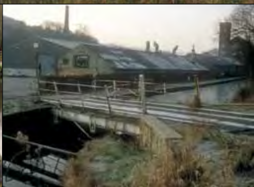
Holme Mill swing bridge, Golcar, in 1998. The upper, fixed deck was added in the 1920s.
