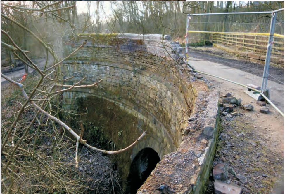
Below: Damaged parapet at Valley Aqueduct
