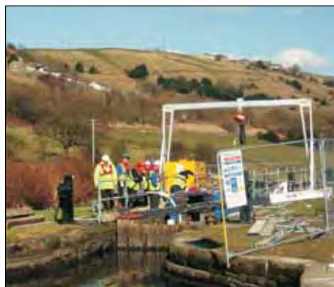
British Waterways staff working to replace the lock gates at Lock 31E, Lingards Wood
