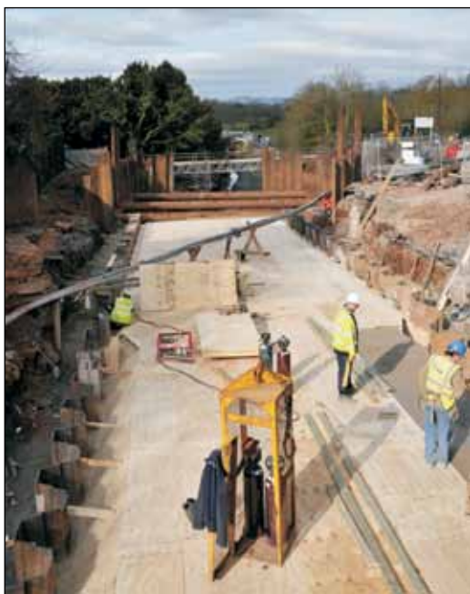
Preparing to cast the bridge at the A449 crossing of the Droitwich Barge Canal.
