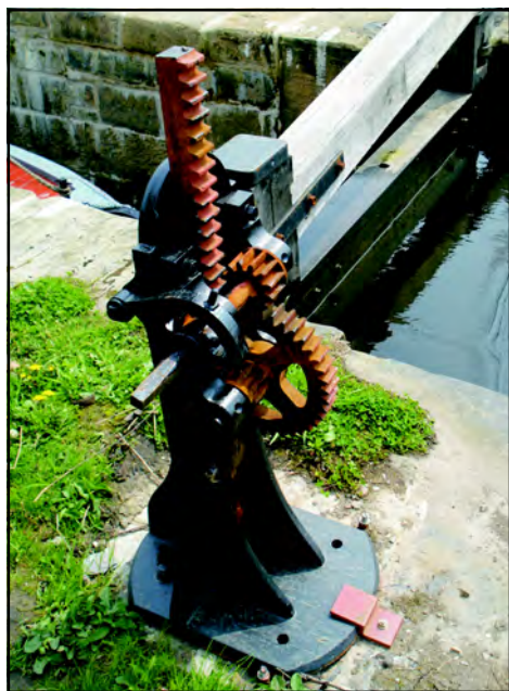
Paddle gear at Lock 10E in need of some TLC (Thorough Lubricating Concoction ....)
