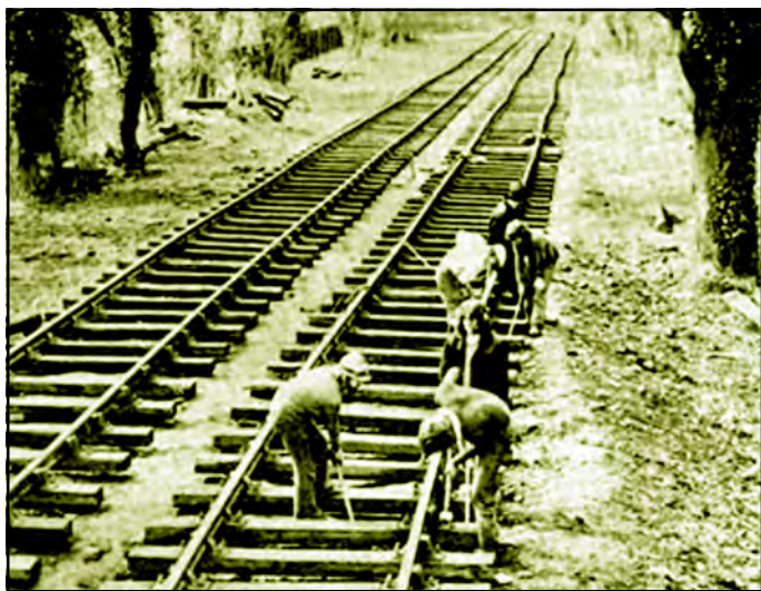
Members of a PFCS Working Party helping to replace the rails on the Hay Inclined Plane - April 1975
