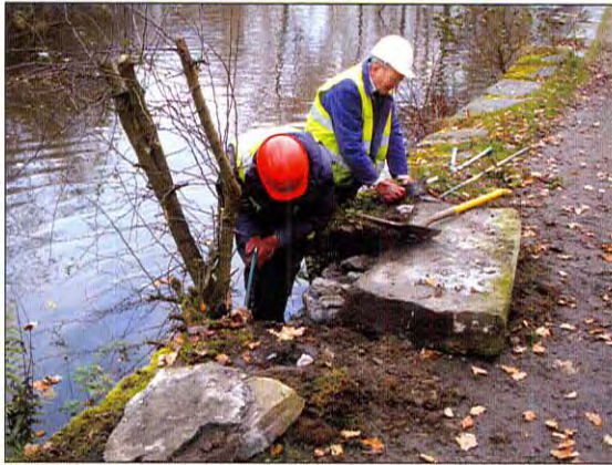
Removing a tree stump from towpath edge
