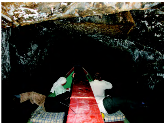
A pair of leggers working an unlined section.
