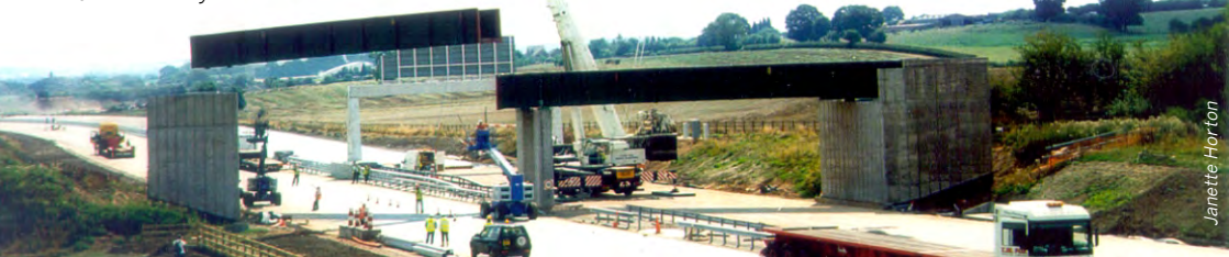
Installing the new aqueduct for the Lichfield Canal over the M6 Toll motorway
