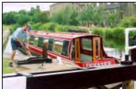
Handspike operated gearing - Calder & Hebble
