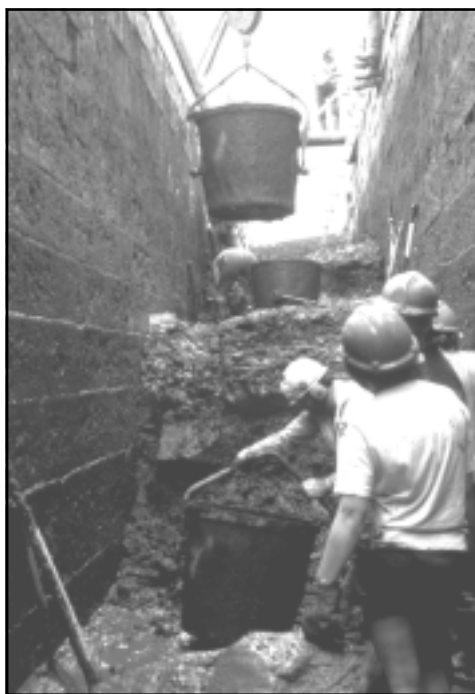
Fig. 6. Early Restoration of a lock on the Huddersfield Narrow Canal (Courtesy of R. Dewey, Huddersfield Canal Society)
