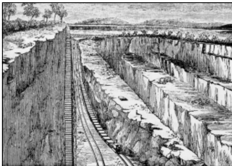
The original (French) Corinth Canal company at work. Cutting is being done in a series of levels, spoil being loaded into small tipping wagons which are run by inclined plane to the lowest level, 5ft above the sea. There they are pushed by locomotive to a heavy steam dredger and lines of barges. These last, when loaded, are taken out to sea to be emptied. (Hadfield, C., 1986, World Canals, David and Charles)
