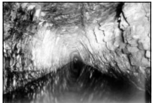
Fig. 8. An unlined section of the Standedge Tunnel (Courtesy of Huddersfield Canal Society)
