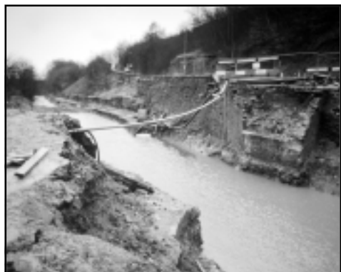
Below Left: The old Lees Mill bridge has been removed and dams formed to allow pumping out of the short length of canal. The dam in the distant right carries the diverted farm access and bridleway. The temporary fencing is suffering in the high winds.
