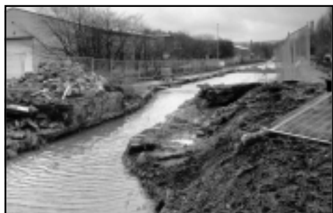
Below Right: The excavated Golcar Aqueduct with the top of the arch visible on the right. Either side of the arch, concrete has been poured to start the 'saddle'.
