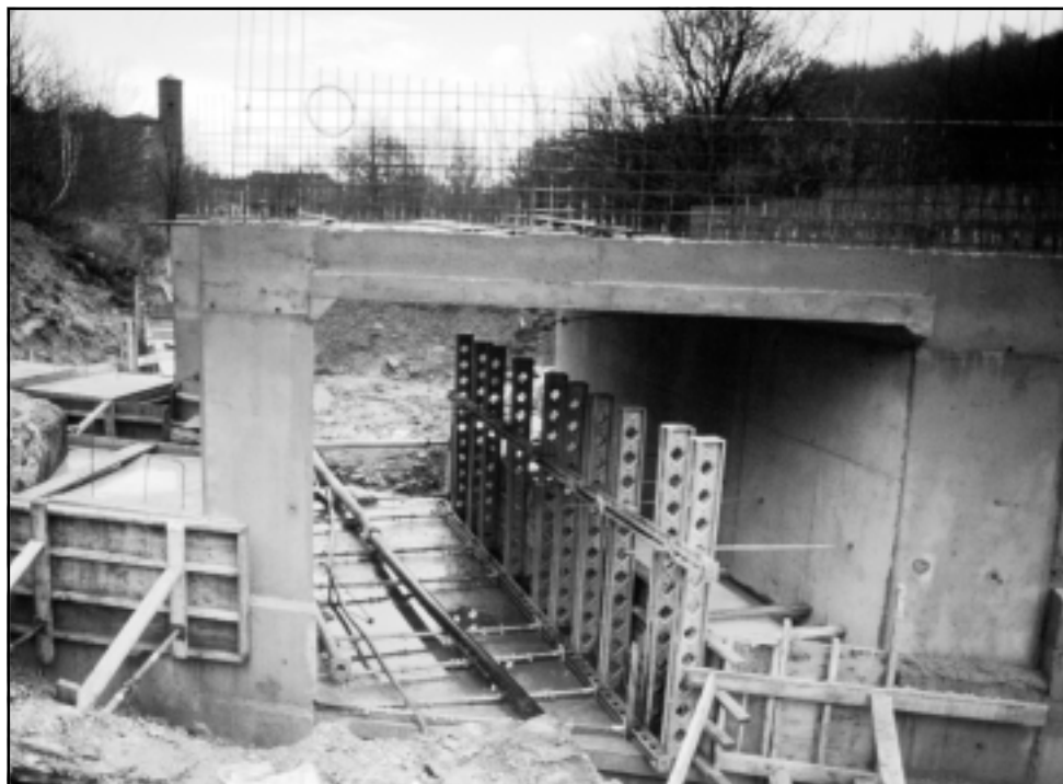
Above Left: The new Holme Mill Bridge with the basic box culvert complete and formwork erected to cast the integral towpath.
