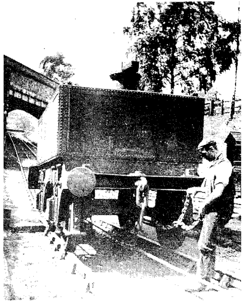
The former Cromford and High Peak Railway was noted for its inclines. These two photographs show wagons at the top and bottom respectively of the 1 in 8 to 1 in 9 Sheep Pasture incline. The wagons were hauled up the incline on a cable to which the wagons were attached.
