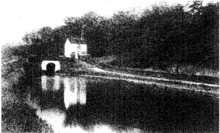
LOCK HOUSE, STALYBRIDGE.
