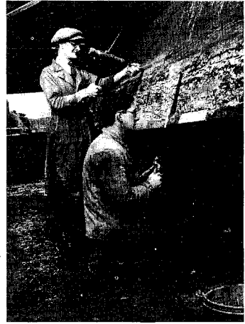
Tooley's yard at Banbury. George, left, is caulking seams with oakum and grease. Herbert, right, is fitting a new elm bottom plank.
