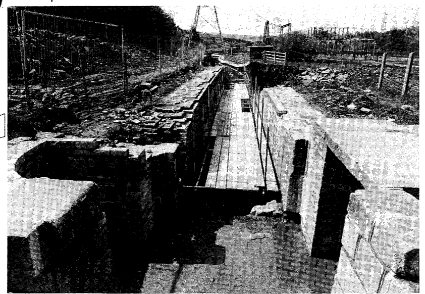
Work in progress rebuilding Lock 8W at Heyrod.
