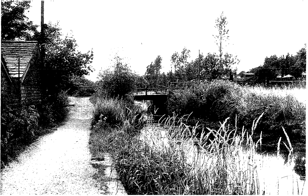
Lees Mill, Slaithwaite. A very low accommodation bridge, to be replaced by a typical canal lift bridge.
