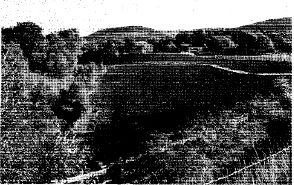
The embankment adjacent to Lock 12W has been removed and the resulting landscaping works blend well into the local topography.
