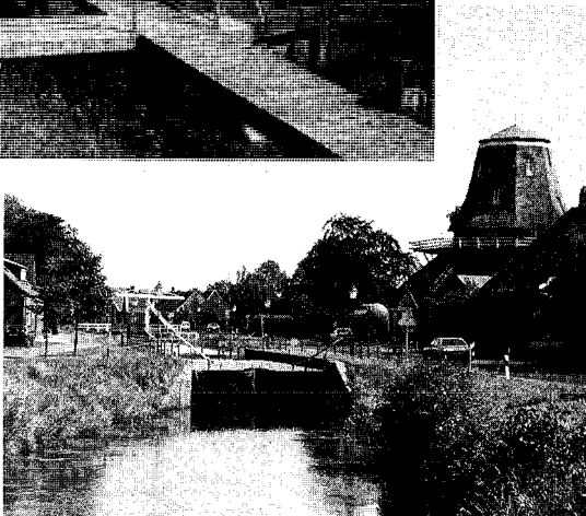
Right: Picture - 2 Lock No.5 (below MSL) note the landscaping and the distinctive lanterns alongside lock and canal
