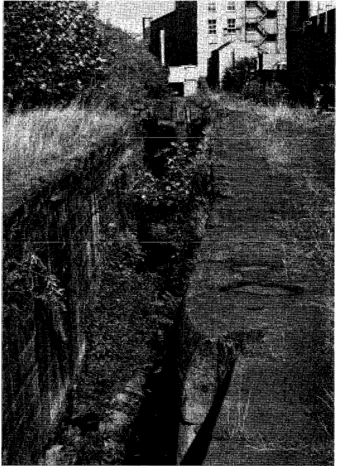
Lock 2E, Huddersfield; major reconstruction work is called for. Note the old lock gates at the tail end. Photo: A. Ogborn
