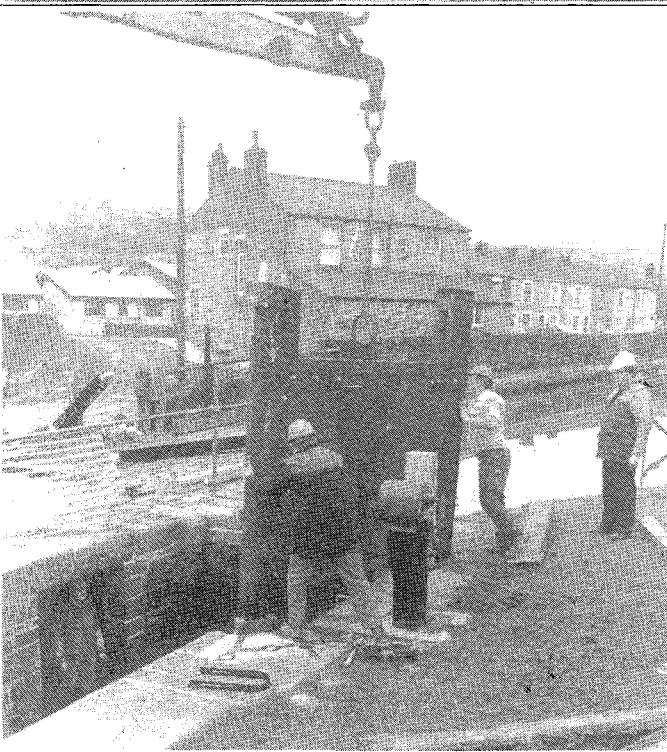
The top gate being swung into position, with Steve Whitby giving it a Paddington hard state to make it fit correctly.
