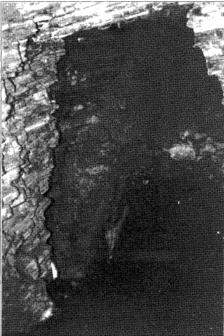
PLATE 81 Ch. 3669 – Ch. 4043 Grindlow shales. Unstable sections will require full lining and rock bolting with mesh and gunite.
