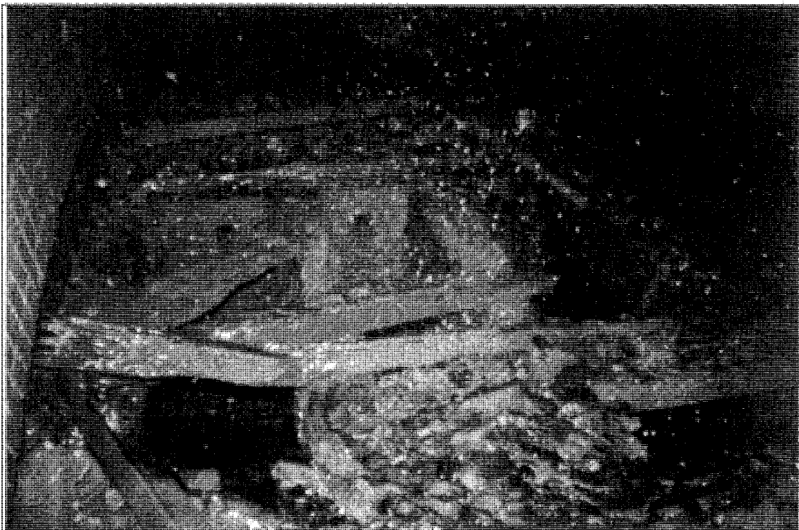
PLATE 41 Base structure, Pule Ventilation Shaft, 141m below ground level.
