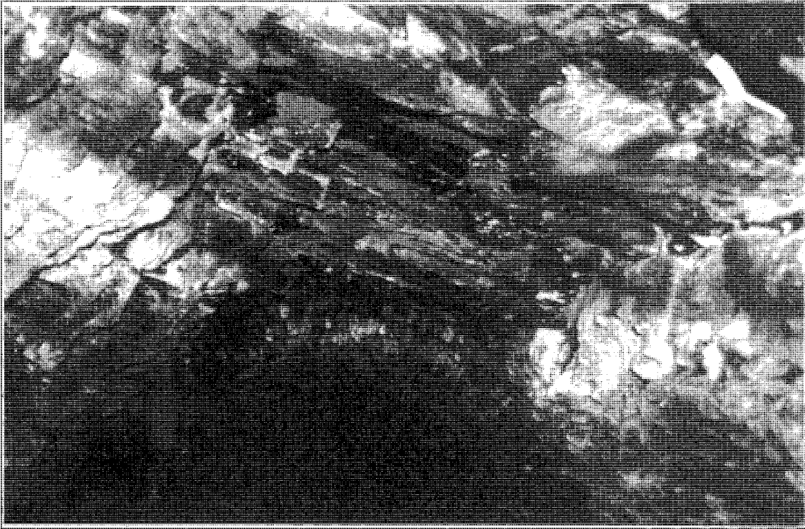
PLATE 81 Ch. 3669 – Ch. 4043 Grindlow shales. Unstable sections will require full lining and rock bolting with mesh and gunite.
