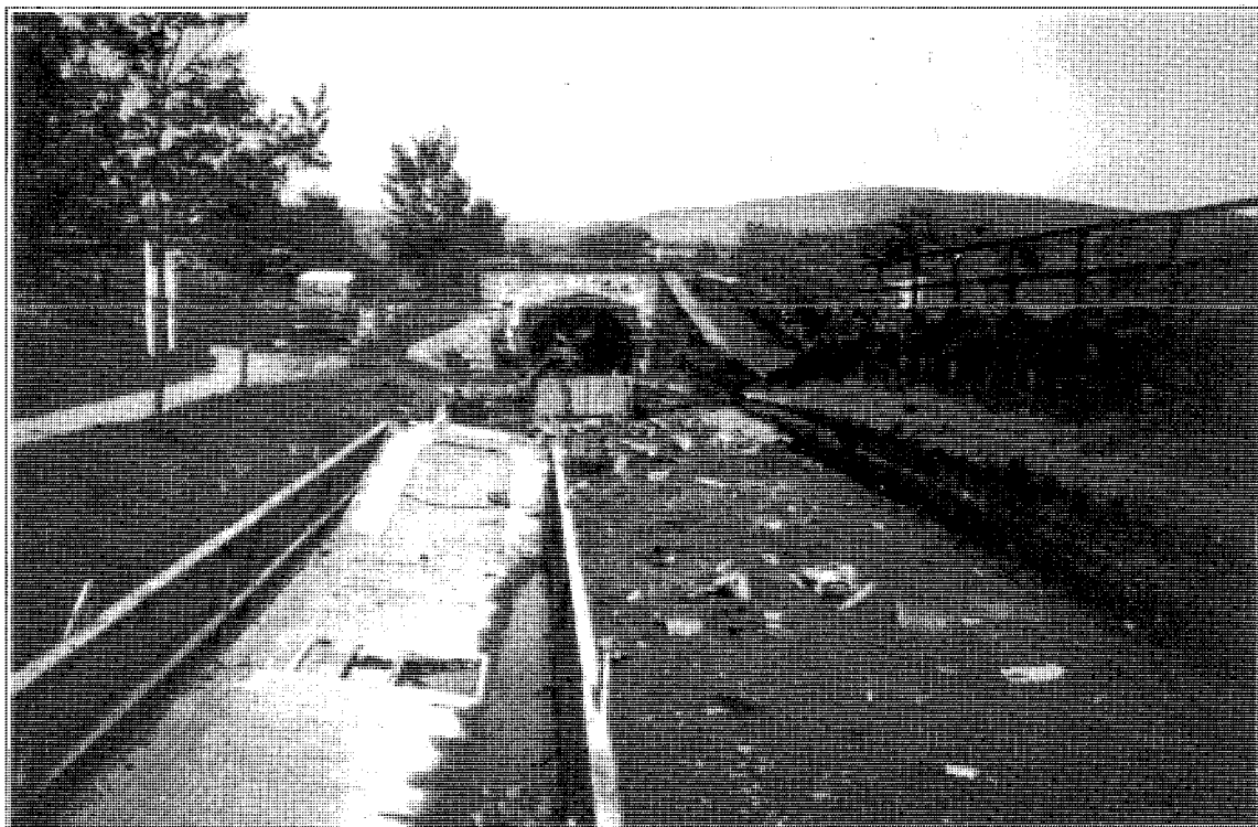
PLATE 29 Diggle Portal and Canal Basin after de-watering had taken place
