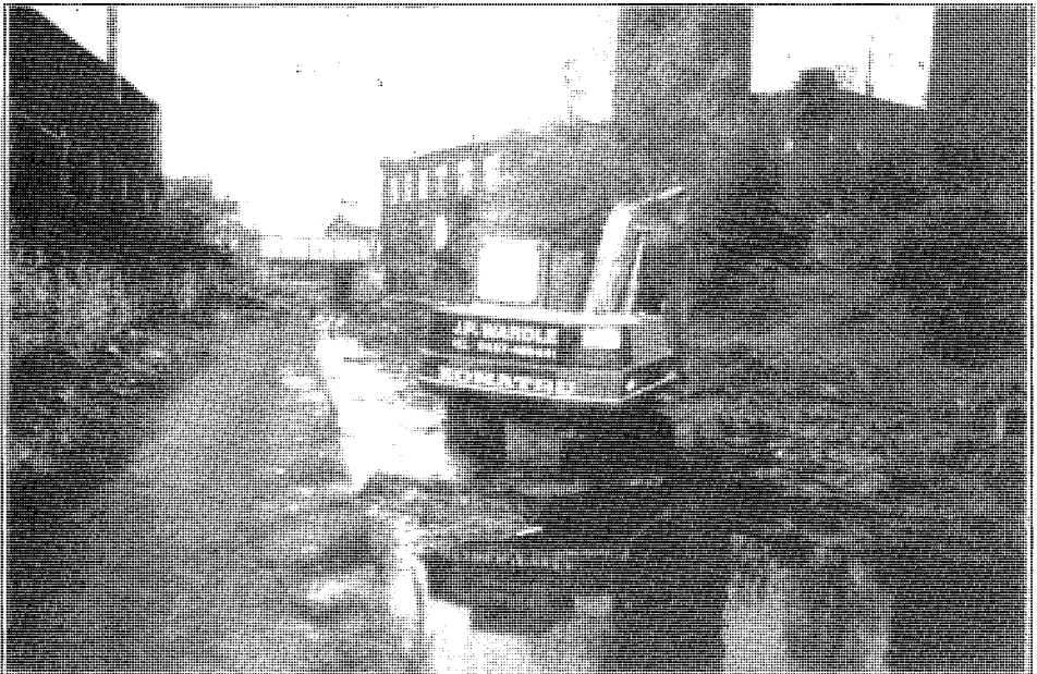
Dredging in progress near Stamford Group Mill
