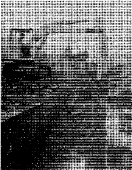
Excavator hard at work at Lock 32W. Photo: Trevor Ellis
