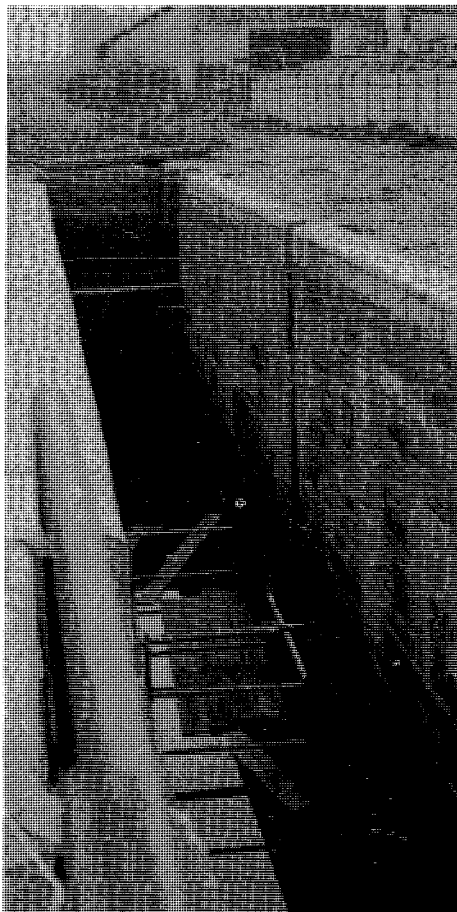
Photo 5: The rebuilt walls of Lock 3 West.
