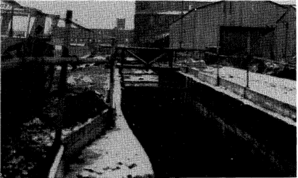
Lock 1 West after the removal of the concrete cap and crushed stone infill. The concrete plug at the tail of the lock (under the temporary footbridge) remains to be broken up and removed before restoration of the walls can begin.
