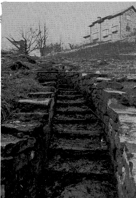
The by wash to Lock 35E. (photo: Kathryn Goodwin)
