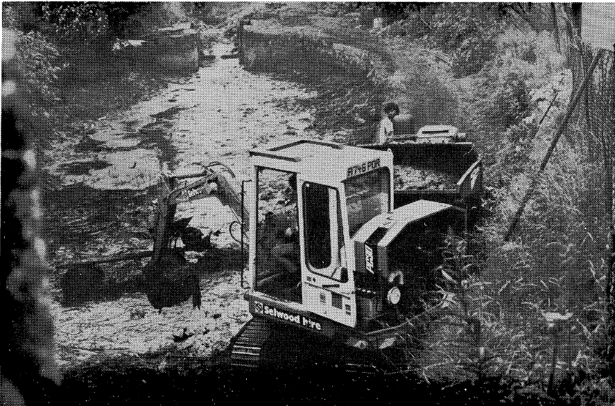
Dredging the pound between Locks 38 and 39 East. A view from the bridge at Warehouse Mill looking towards Lock 38E.
