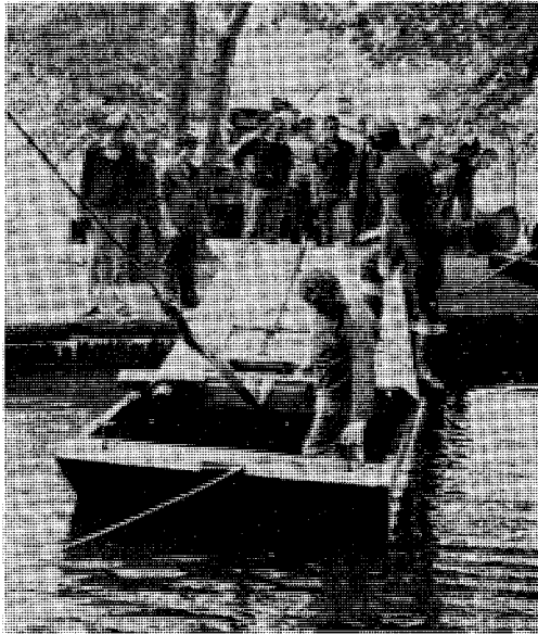
Photo shows a lockgate being manoeuvred onto the work punt.
