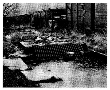
Lock 74 (1W) showing infilled lock chamber.
